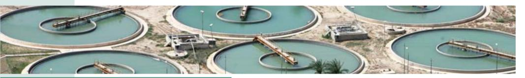
The Raw Water Treatment sub-series discusses Sedimentation, Clarification and Disinfection, processes which are an essential part of raw water treatment systems.
